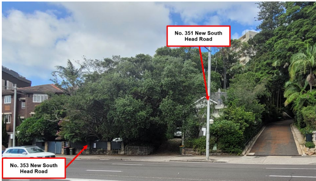
View of the subject sites from New South Head Road
